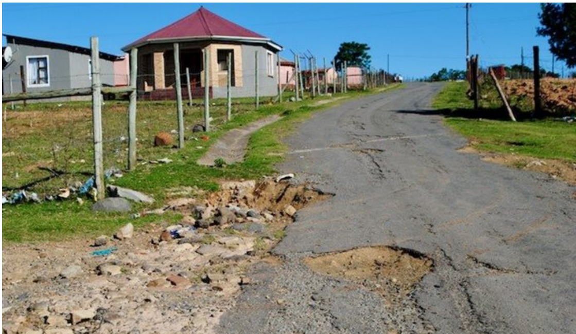
The tarred access road in Lwalweni that “Madiba built” is potholed, cracked and not maintained. | Photo: Mkhusele Sizani
