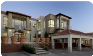
Clearwater Office Park
