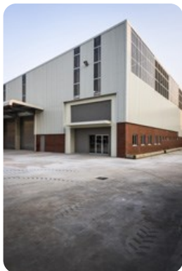
CHC Resources warehouse in Durban's Prospecton node.
