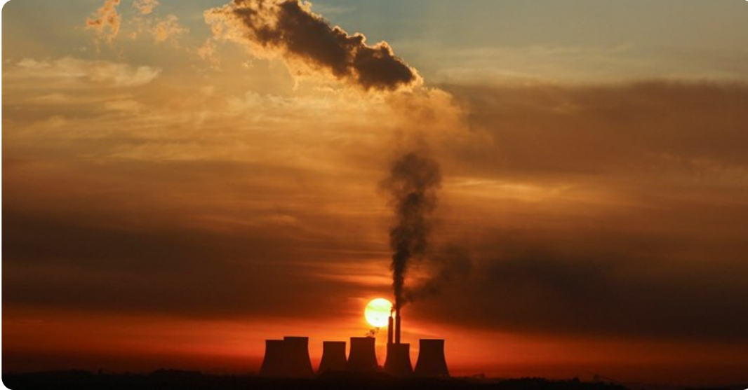
Sun rises behind the cooling towers of Kendal Power Station, a coal-fired station of South African utility Eskom, as the company's ageing coal-fired plants cause frequent power outages, near Witbank. Source: Reuters/Siphwe Sibeko
