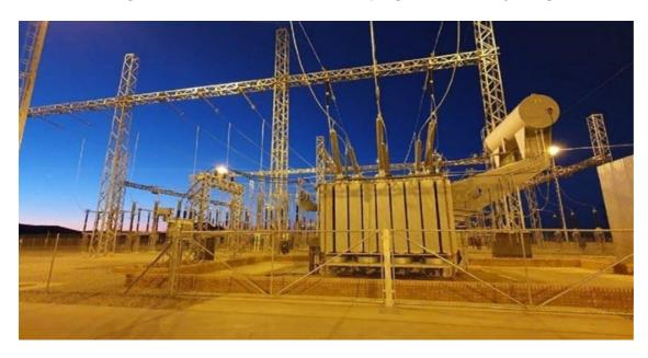
The 250MVA transformer is locally manufactured and arrived in the Northern Cape via road from Gauteng last week. Housed at the Groeipunt Transmission substation, the transformer receives generated power from the wind farm via a distribution network, where it is responsible to step the voltage up from 132kV to 220kV.
