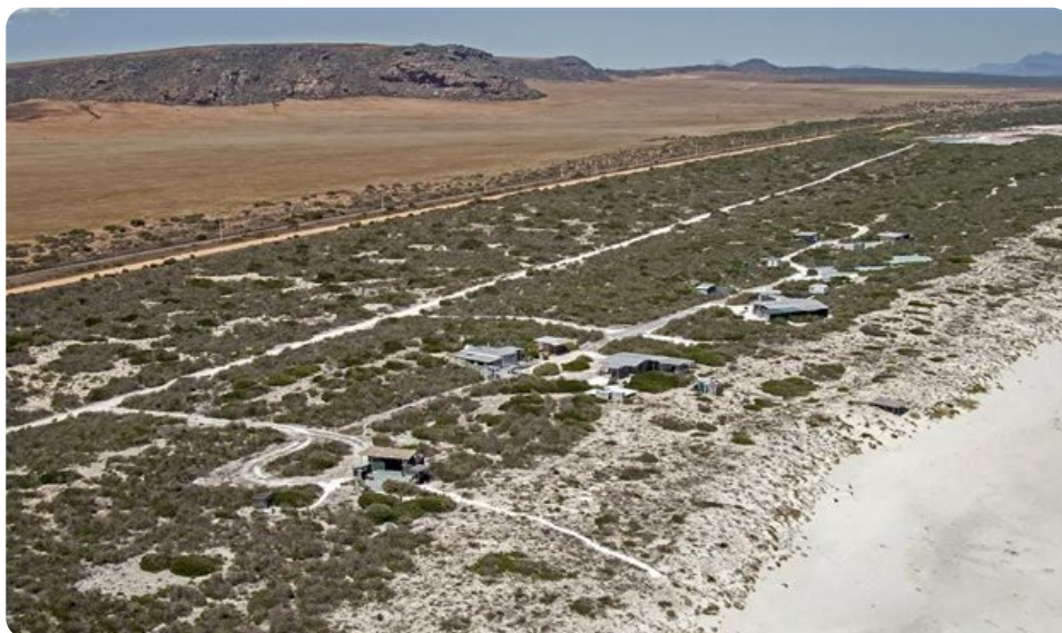
Some of the structures at a private nature reserve on Mosselbaai Farm south of Elands Bay on the West Coast. The Western Cape government had instituted legal action for alleged environmental contraventions by some owners – including building too close to the beach.
