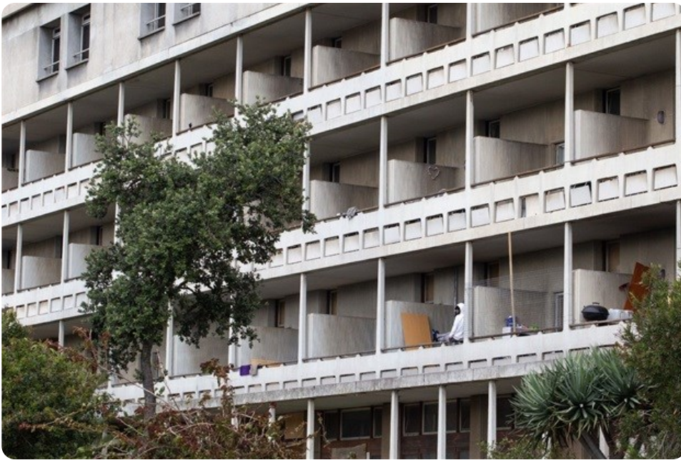
Helen Bowden Nurses Home has been occupied by social housing activists since March 2017. The Western Cape government has now been given the go-ahead to develop the area for affordable housing. Photo: Ashraf Hendricks
