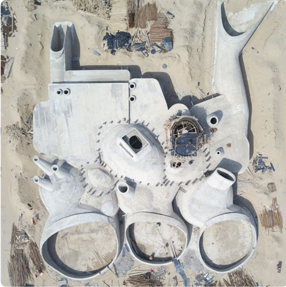
UCCA Dune Construction. Image © OPEN
