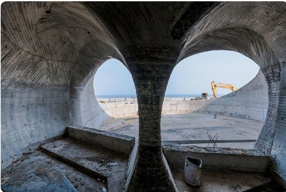
UCCA Dune Construction. Image © Ni Nan
