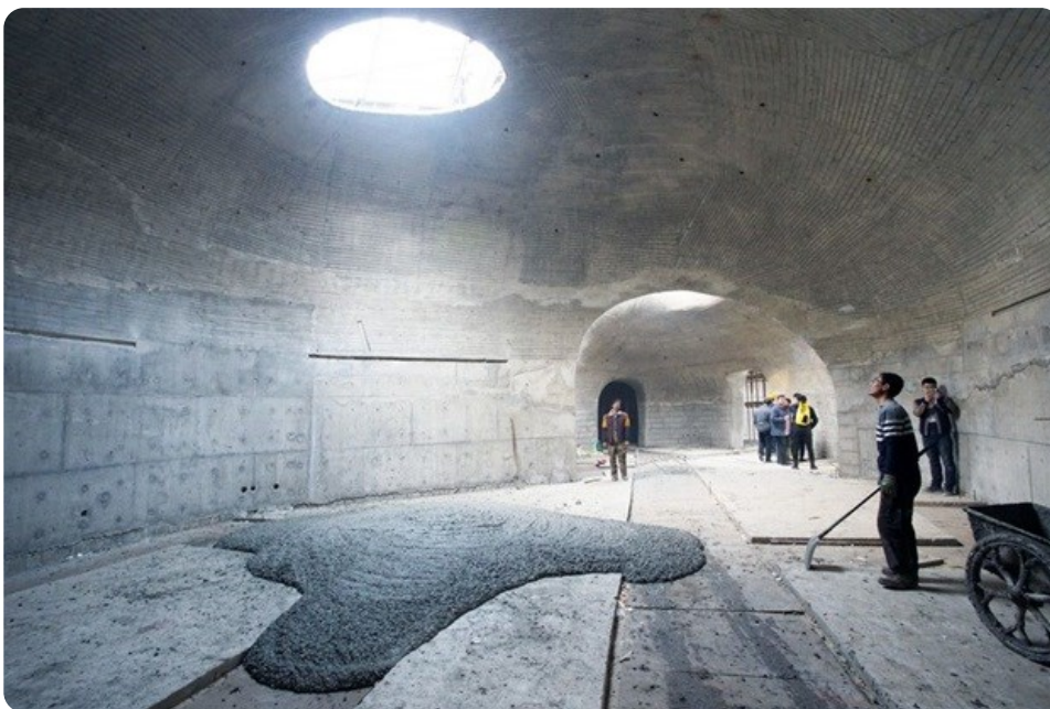
UCCA Dune Construction. Image © OPEN
