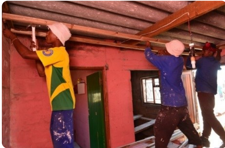
General Vrygrond project archive photo: a ceiling being retrofitted.
