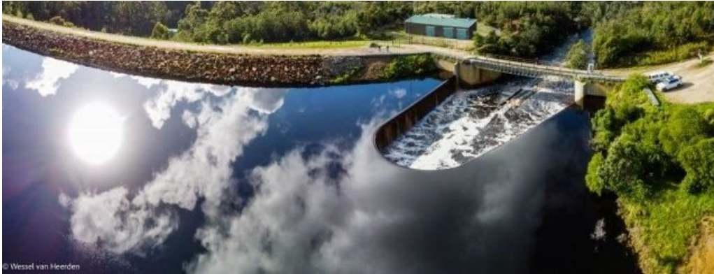
Zutari designed the duckbill-shaped spillway to slow down water flow using basic physics principles. Image: Wessel van Heerden
