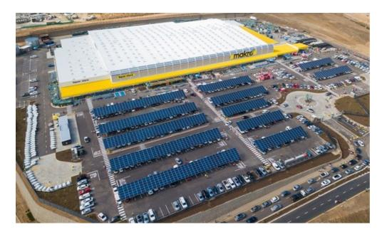
Makro Strubens Valley in Gauteng became the sixth Massmart store to make use of renewable energy. The store has a 480 kilowatt (kWh) peak plant that consists of 147 car park-mounted polycrystalline PV panels. The plant provides nearly half of the store's daily energy requirements and is estimated to provide 24% of the store's total annual energy consumption.
