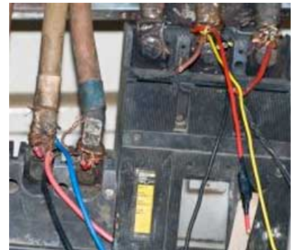
Illegal electricity connections pose dangers to the community and can damage Eskom's power grid. It is a criminal offence to make illegal connections and steal electricity. Image: Operation Khanyisa
