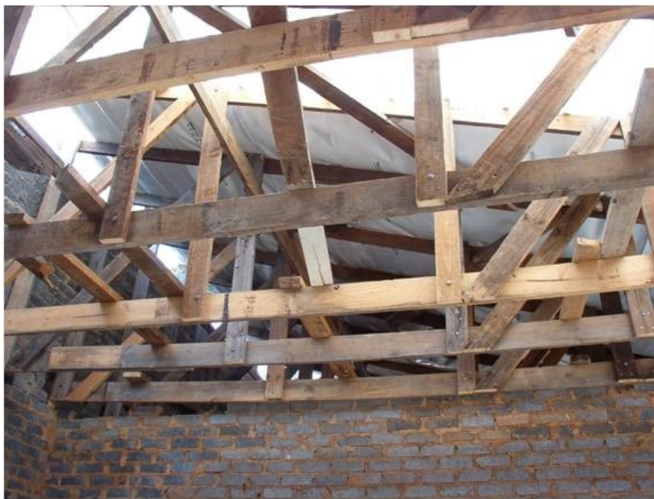
An example of a site-manufactured roof structure that will threaten life and limb.
