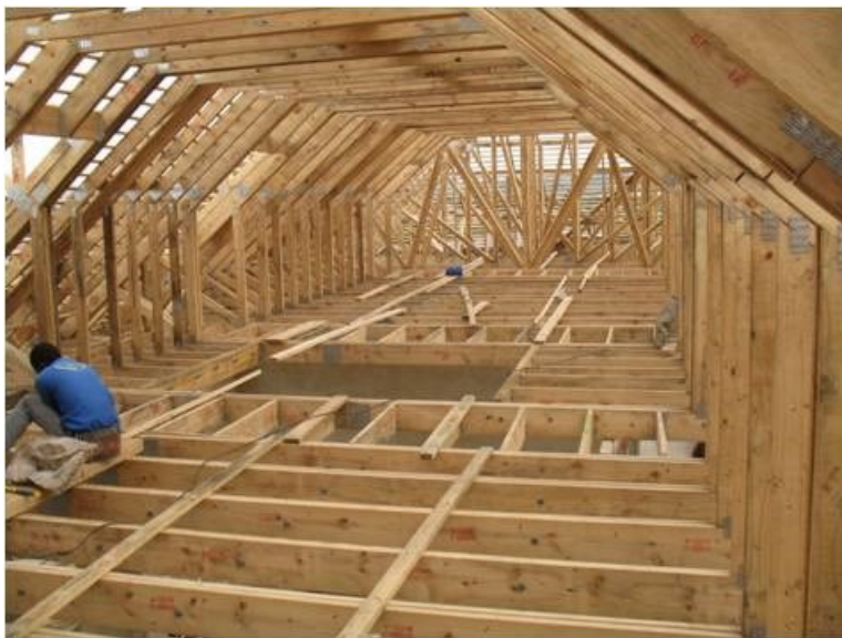
A fully compliant roof structure as manufactured by a professional member of the ITC-SA. (Image: MTEK Industries SA)
