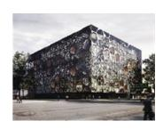
Michel said despite initial reservations from the client the ADD process played an integral role and allowed Rojkind Arquitectos to design a beehive-like, porous facade made of different sized hexagons in fiberglass, steel, aluminium and glass that would expand the envelope of the building to create the space required.
